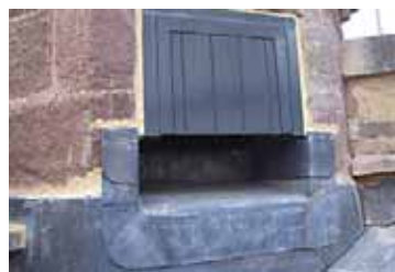
External mitigation at Ashton Court
